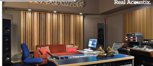
Rear diffusers and open ceiling construction help create a reflection-free zone. Inset: Behind the tape machines and racks are FlutterX panels from Real Acoustix.
